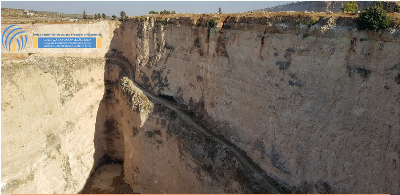
Another picture of Al-Habbat Quarry
